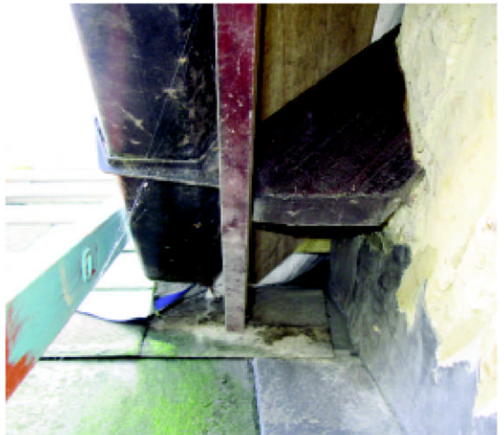
If you look up the side abutment you can see the white underlay and a gap up through which rats and mice can climb.
