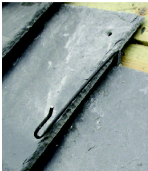
Slate hooks are manufactured in a range of metals, but only stainless steel should be used in the UK.
