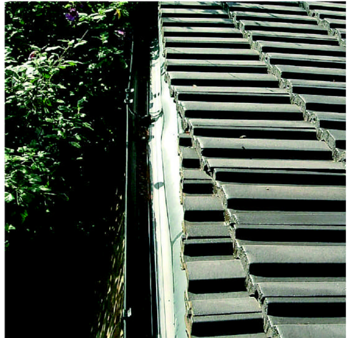
This may look like a raking eaves but it is also a raking verge. Note the step down where the lower course diminishes to nothing, causing the upper tiles to dip.
