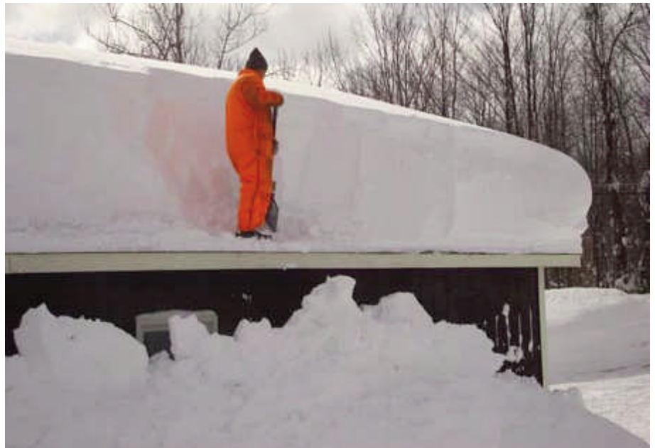
'Installing a house designed for southern Spain (with a shallow pitch roof) in a mountainous region, may not be a good plan'
