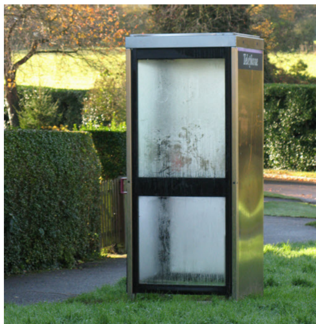
An unheated telephone box running with condensation
